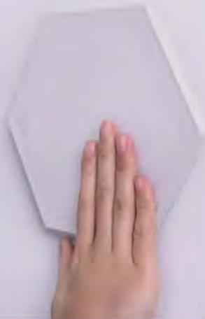
Press the panel to the wall for 30 seconds
